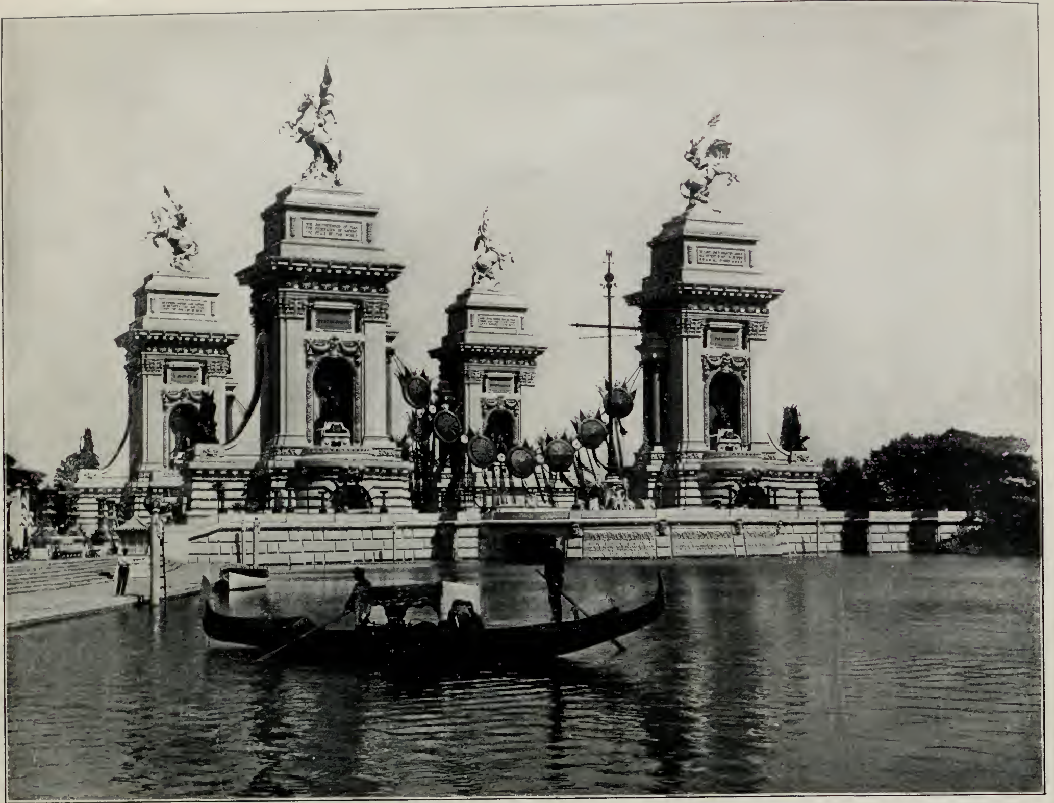
TRIUMPHAL BRIDGE FROM THE MINES BUILDING
